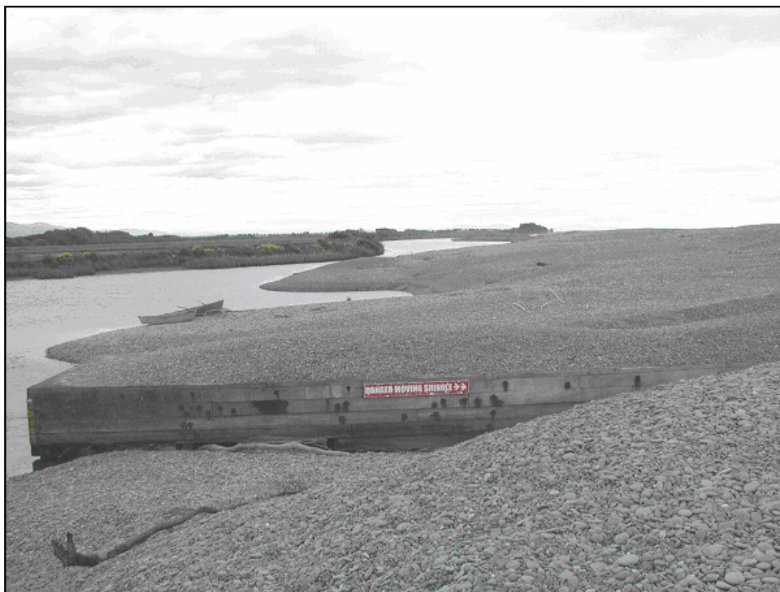
Figure 5.3 Entry to the Waihao Box looking north along the Dead Arm
