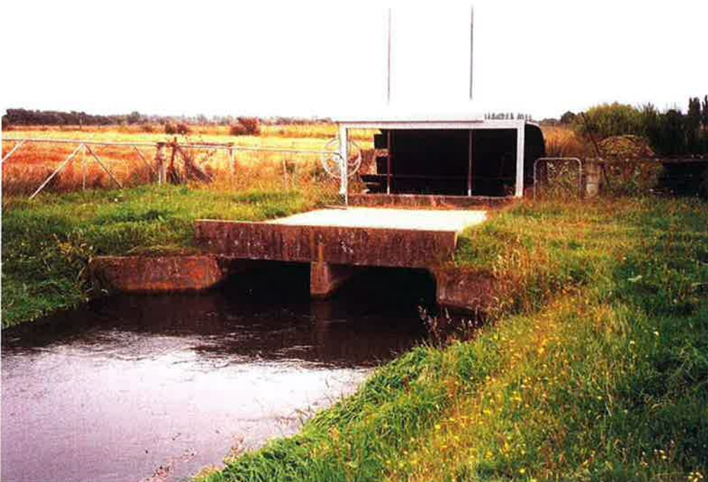
Figure 5.11 Greenstreet Irrigation Scheme intake and fish screen, 911 \text{ l s}^{-1} , 29 th February 2000.
