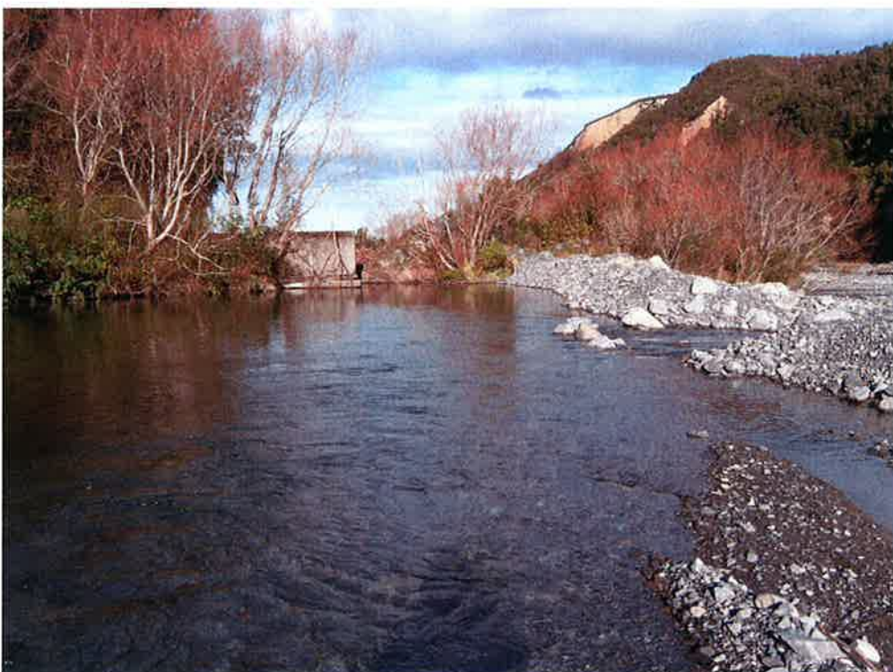
Figure 5.9 Pudding Hill intake. 4 th June 2003. Abstracting approximately 380 l s -1
