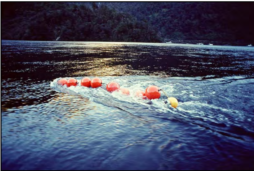
Figure 6: Tailrace flow at 650 m 3 /s
