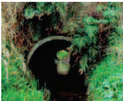
A well designed culvert allows fish access upstream
