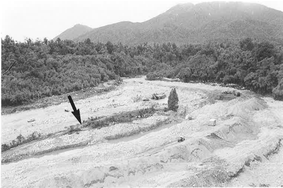
FIGURE 2. Thames Minerals Ltd. concession on the Big Hohonu River, August 1987. Visible are an excavator and dredge (centre); untouched river channel (indicated); dredge ponds; stockpiled fines for re-distribution after mining ended; and (bottom right, curving into the centre immediately in front of the bush line) the excavated channel to carry the diversion.
