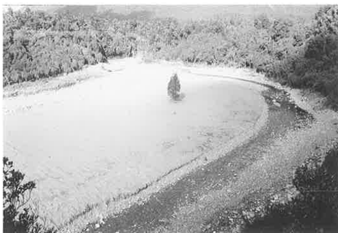
FIGURE 11. The Big Hohonu River Diversion, September 1988. The stream has reverted to the true right of the channel and is generally much broader than formerly.
