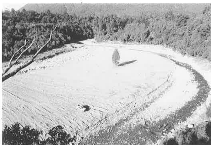
FIGURE 10. The Big Hohonu River Diversion, June 1988. The stream has shifted to the true left of its channel, but also has eaten away at the right bank.
