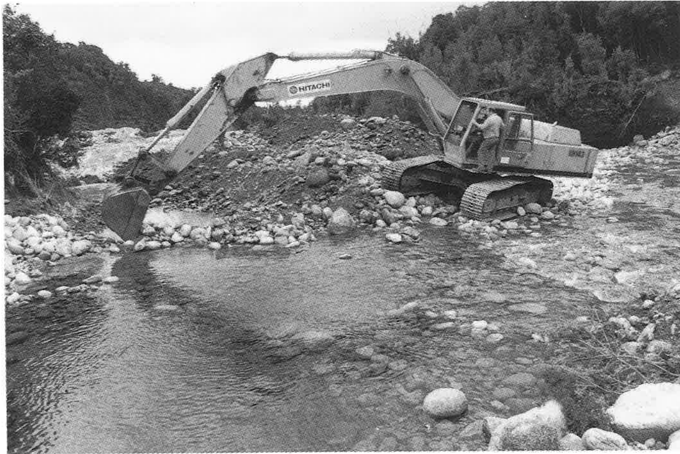
FIGURE 5. The diversion of the Big Hohonu River being cut, August 1987. The new channel was cut at a lower level than the stream. This allowed the diversion to take place without any sediment entering the old channel, and facilitated the salvage of fish from the residual water.
