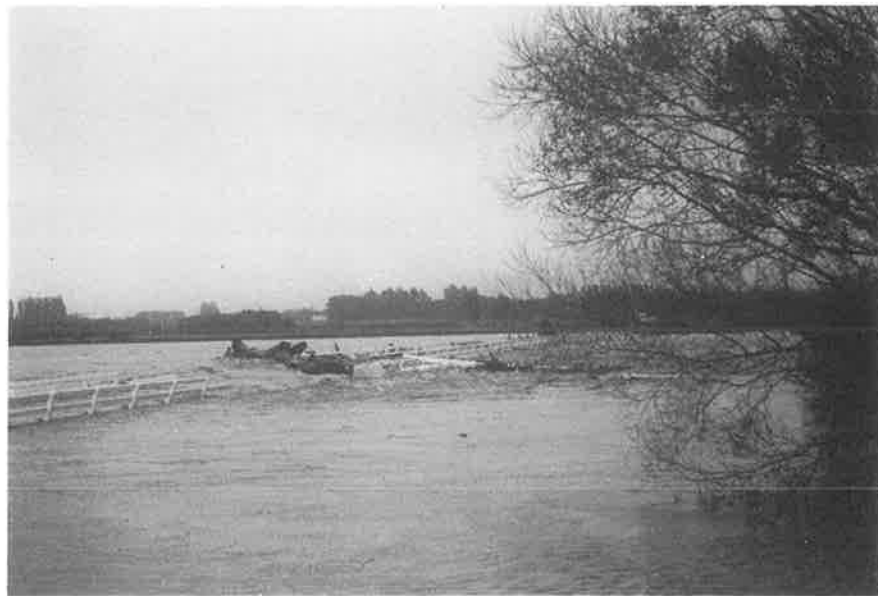
Bradshaws Bridge on Waihao River. Flood debris demolishing the handrails. (Courtesy M.E. Bruce).
