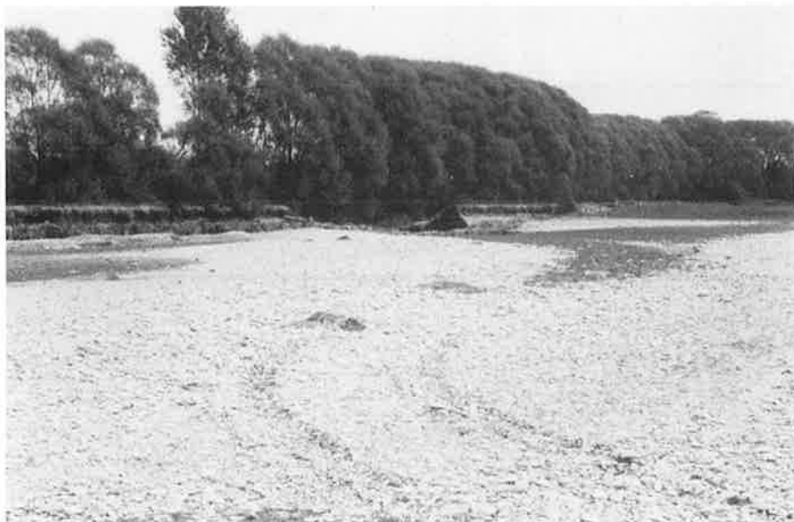
Shingle deposited onto farmland carried by flow through the breach in the stopbank (mid photo).
