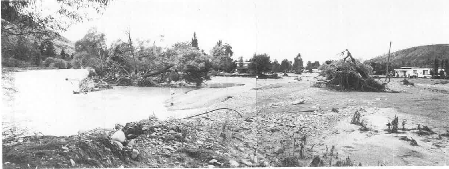
Overtopping and subsequent breaching of the stopbank at Pareora Huts caused major damage to buildings, roads and services in the area.
