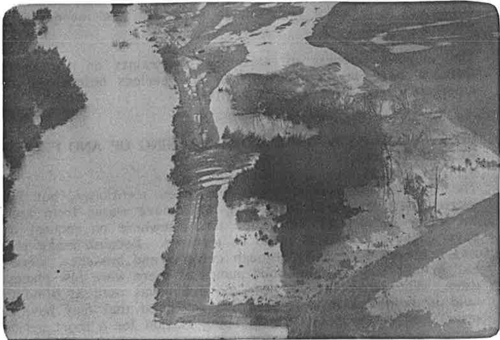
Fig. 13. Failure of a river training bank with the flood control stopbank to the right. (Monday).
