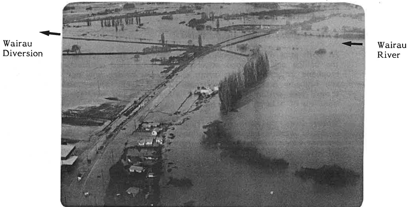
Fig. 7. Stopbanks overflowing at Tuamarina. The Wairau River and road and rail bridges in the background.
