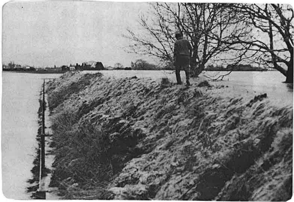
Fig. 6. Typical overflow in the Lower Wairau River. Some overflows were 0.3m deep.
