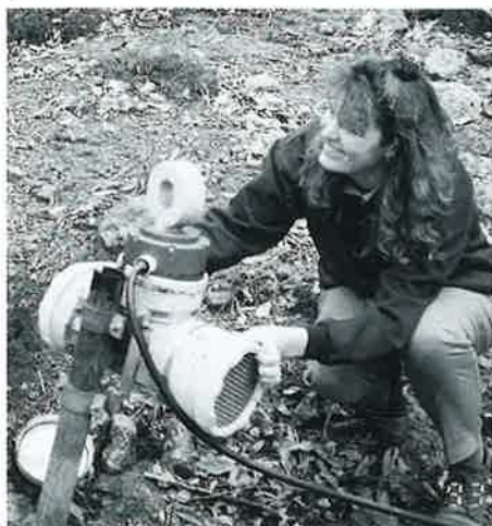
Real-time monitoring salinity unit – South West region.
