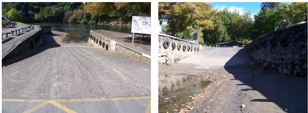
Figure 1: Roose Commence Boat Ramp (Hamilton) - BECA.
