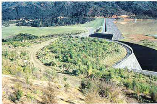
The same site as above in April 1974. Only native species were used to revegetate the site. Photo A. Dakin.
