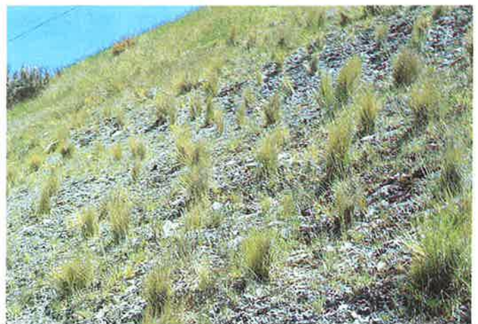
Road batter stabilisation in central Otago using Festuca novae-zelandiae . Photo J. S. Sheppard
