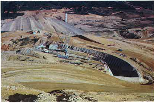
Mangatawhiri dam site, Hunua, at time of construction, 1970. Photo A. Dakin.
