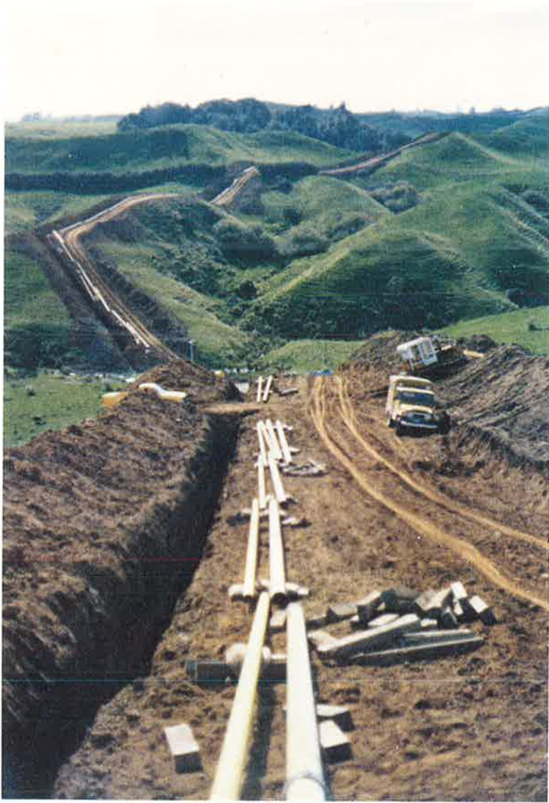
Figure 2: McKee oil lines near New Plymouth, 1984. Note the stockpile of topsoil on one side and trenching material of subsoil on the other, with the trench and the right-of-way between. Access to the right-of-way is had by leaving a gap in the stockpile of subsoil and a plug in the trench.
