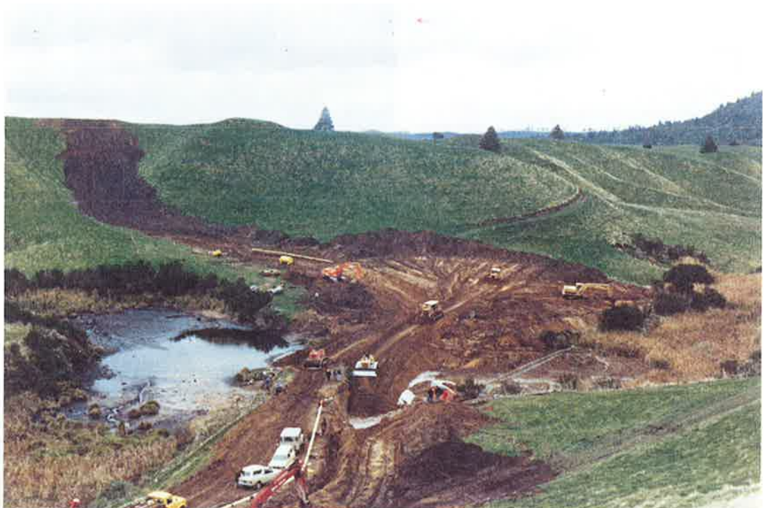
Figure 3: Kinleith—Kawerau natural gas line, 1982. At problem points, such as stream crossings, extra working areas must be allowed for. If they are not, then stripped topsoil may be lost and restoration become difficult.
