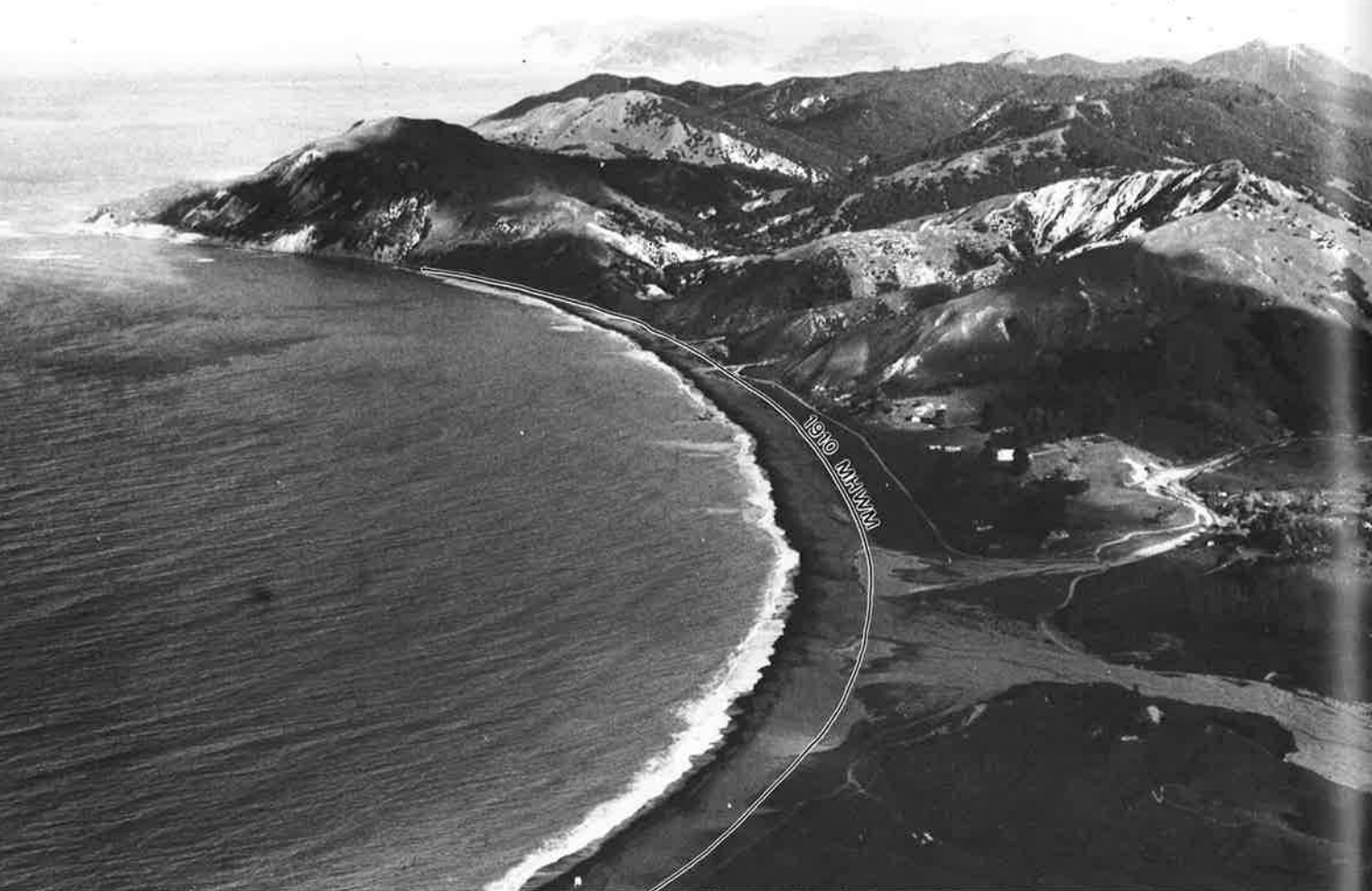
Figure 9 Oblique aerial view of Tuparoa looking south. The 1910 shore line position is shown and indicates about 50 m of accretion from bedload supplied by the Tohoratea River, Waitekaha Stream, and two unnamed streams about 1 km south. Note the extensive aggradation in the Waitekaha Stream bed, foreground. [21 May 1979]
