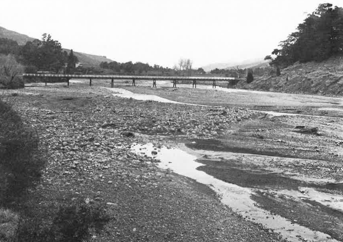
Figure 7 The bridge over Tapuaeroa River bed, looking downstream. Pahikiroa Station is on the right. From 1912 to 1979 the river bed has aggraded 13.72 m under the bridge. [25 June 1980]
