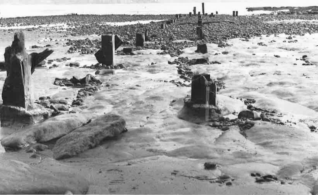
Figure 15 Looking west across Kawakawa Bay towards Matakaoa Point, showing decapitated wooden wharf piles exposed at low tide on the shore platform plane cut in Late Tertiary rocks 400 m east of Te Araroa. In 1914 the platform plane was level with the concrete around the piles in the foreground. Gravels on the lower plane are from the Awatere River. Plastic rule against the righthand pile is 0.4 m long. [23 May 1979]
