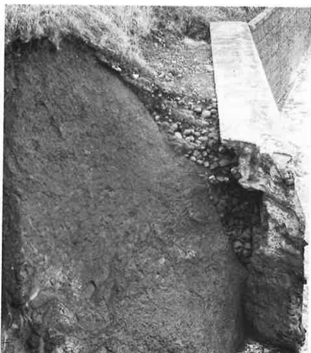
Figure 18 Northern Tokomaru Bay looking north, showing an outflanked sea wall. The rocks are Late Tertiary sandstone-siltstones that have retreated about 7 m since 1945. Note the polygonal cracking breaking up the cliff face. [24 May 1979]
